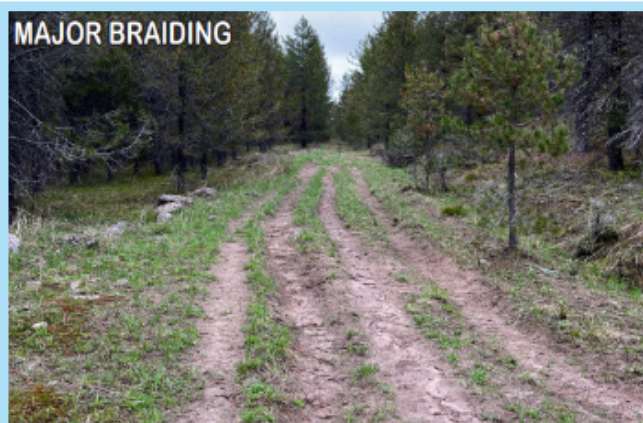
CUPPING / DRAINAGE CAUSING BRAIDING
