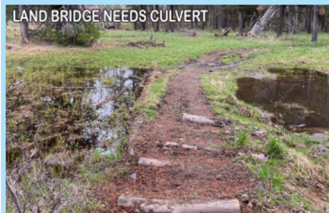
CUPPING / DRAINAGE CAUSING BRAIDING
